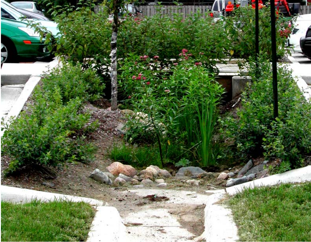
Bioswale in parking lot
